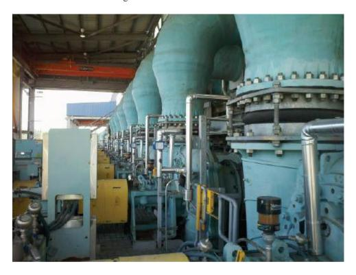
**3. In use.** Expansion joints are used on both the discharge and suction sides of recycle pumps. *Courtesy: Garlock Sealing Technologies*
