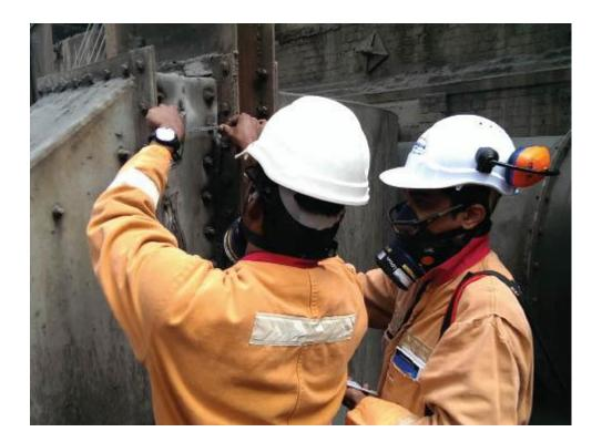
**4. Measure twice, install once.** Measurements before and after installation can detect potentially troublesome offsets. *Courtesy: Garlock Sealing* Technologies
